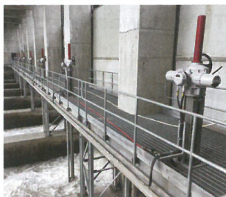
The solution at Forrest Kerr consists of Rotork IQ40 actuators mounted on custom-designed knife gate valves.
